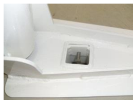
3/8" bolt inside anchor sleeve
